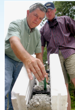
Extension activities encourage the use of energy-efficient, wind-resistant construction materials such as insulating concrete forms (ICFs).
